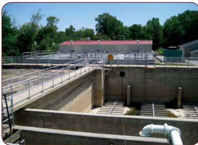
Figure 1: The Village of Dundee wastewater treatment plant installed membrane bioreactor (MBR) technology in 2005, using much of the existing plant, including the conversion of sequential bioreactors (SBRs) to biological process basins for the new system.
